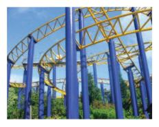
"The Hornet" erected some 10 years previously was showing signs of deterioration on the track and supporting steelwork and without further treatment, the onset of metal fatigue was inevitable.
